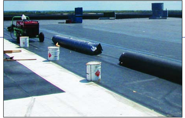
Reroofing project using EPDM single ply membrane.
